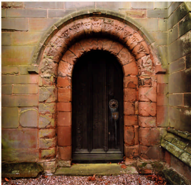
12th century doorway at Northfield church
